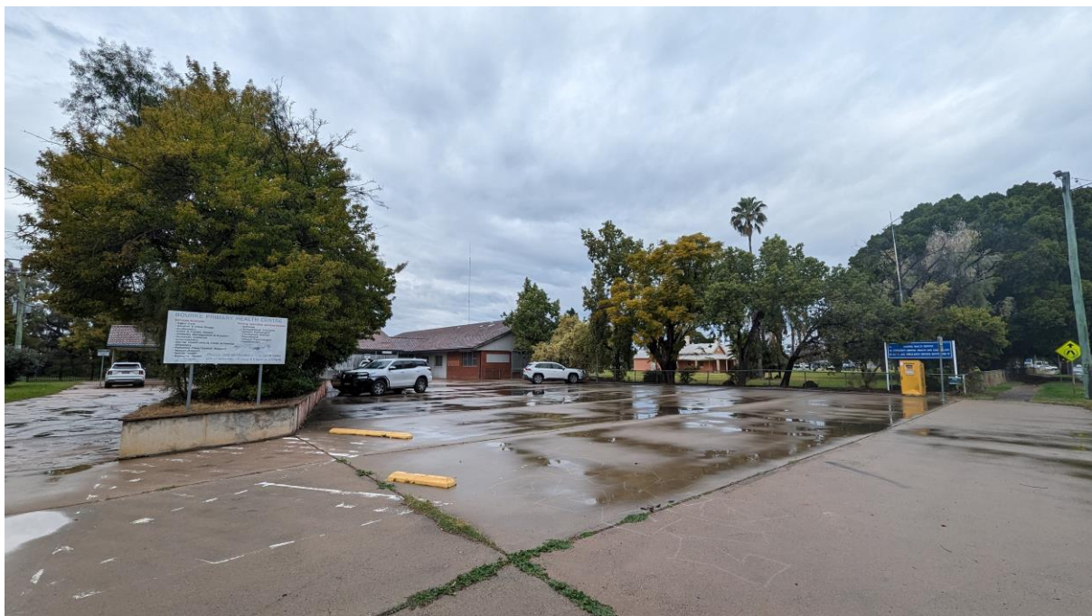
Figure 17 – Bourke Hospital – Tarcoon Street frontage
