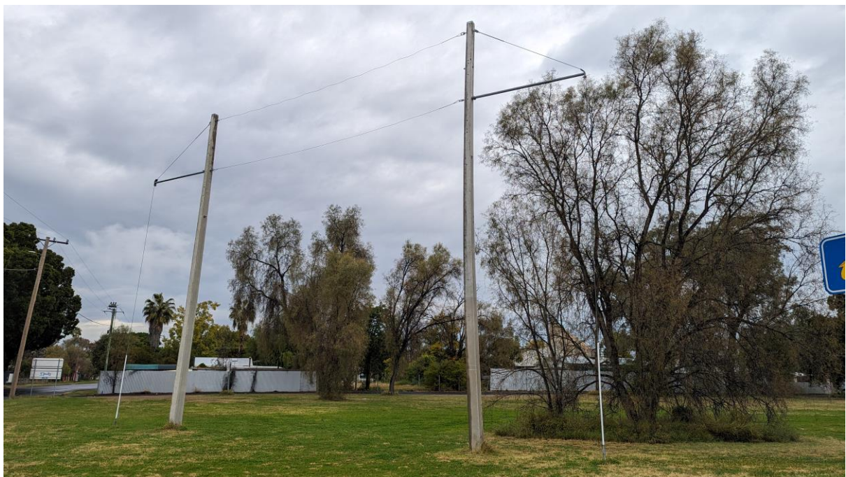
Figure 13 – Poles and stays within the site at the corner of Mitchell and Tarcoon Streets to be demolished
