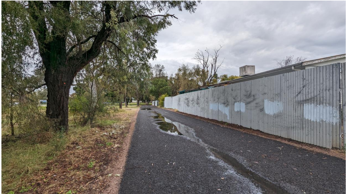
Figure 12 – View of the recently sealed unnamed lane at the rear of the site towards Tarcoon Street
