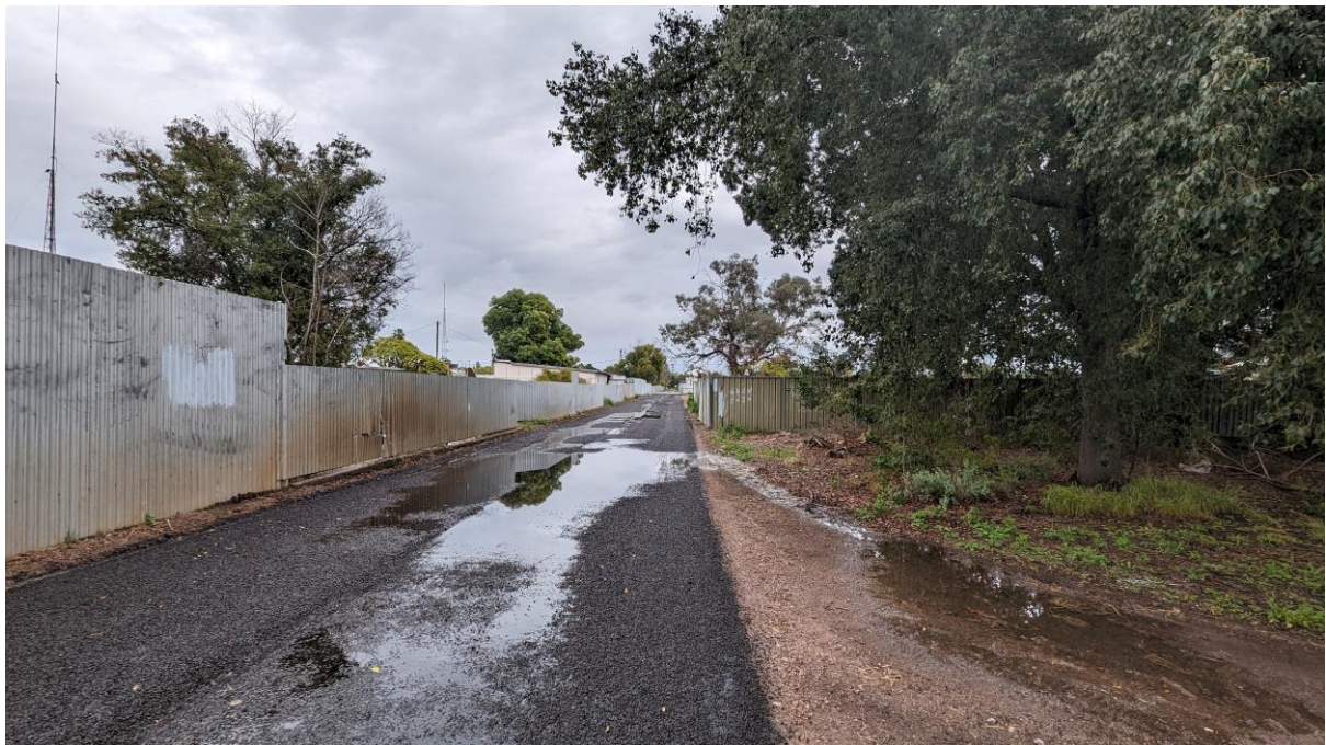
Figure 11 - View of recently sealed unnamed lane to the rear of the site from south-western corner of the site
